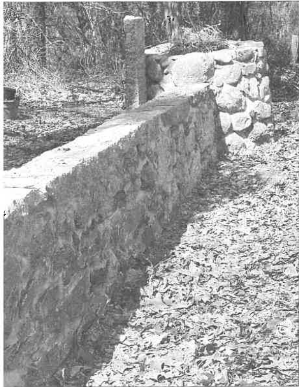
Repointed stone wall at BCT DeNormandie Woods.
